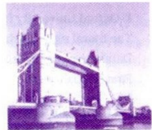
Tower Bridge, London, England
